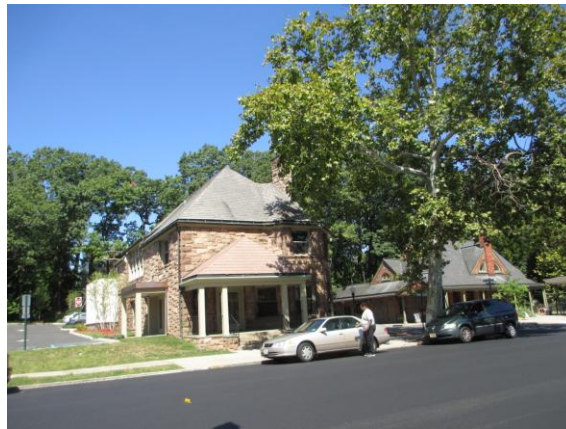
The Boiling Springs Savings Bank on recently repaved Ridgewood Avenue.
